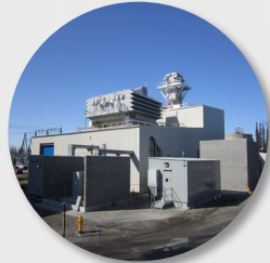
Soldotna Combustion Turbine Plant 48.0 MW
