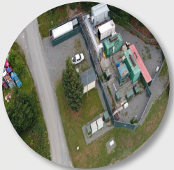
Seldovia Gerry Willard Generation Plant 2.2 MW
