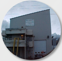
Nikiski Combined Cycle Plant 80.0 MW
